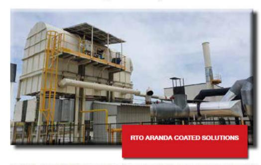
The basic concept behind the design of thermal oxidation is to promote a chemical reaction in the air pollutant with oxygen at high temperatures. This reaction destroys the VOC emission in the air stream by converting it into CO<sub>2</sub>, H<sub>2</sub>O and heat.
